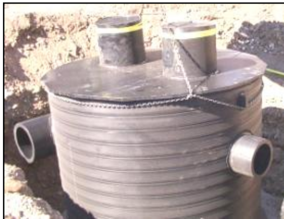
Aqua-Swirl® component of the Aqua-Filter™ System. Note tangential inlet and outlet piping stubouts.
