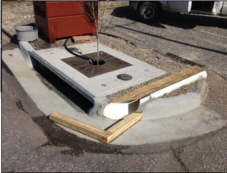
Figure 20. Filterra Site with overflow bypass pipe
