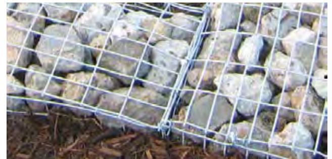
Figure 25: Overfill rock into gabion and seal tight to prevent sagging. Rock will settle over time.
