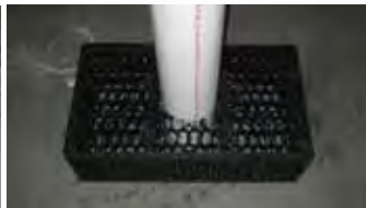
Figure 13: Place inspection port into underdrain module
