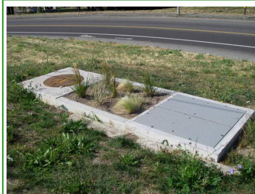
Installation of the monitored Modular Wetland-Linear system at the Albina Maintenance Facility in Portland, Oregon.
