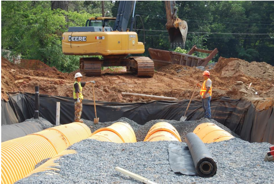
Figure 3: Storm Tech Unit Installation – Photo courtesy of Dan Trask, Storm Tech
