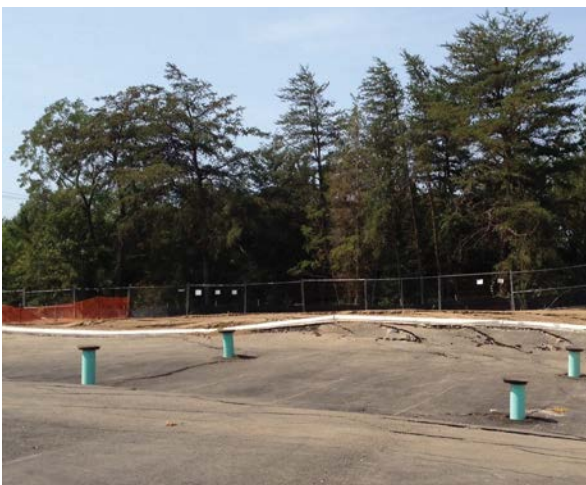
Figure 1: Collapsed parking lot over failed retention system
