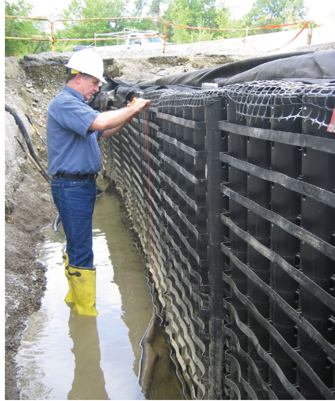
Figure 4: Stackable cellular-type stormwater units
