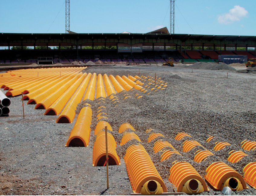
Figure 3: Open-bottom corrugated arched stormwater chambers
