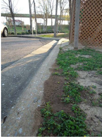
Figure 12 Eroded Ant Hills Adjacent to the Filter Inlet
