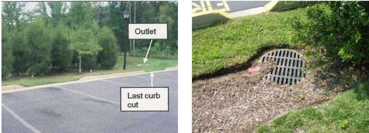
**Figure 9.11. Examples of Short-Circuiting at Bioretention Facilities**
