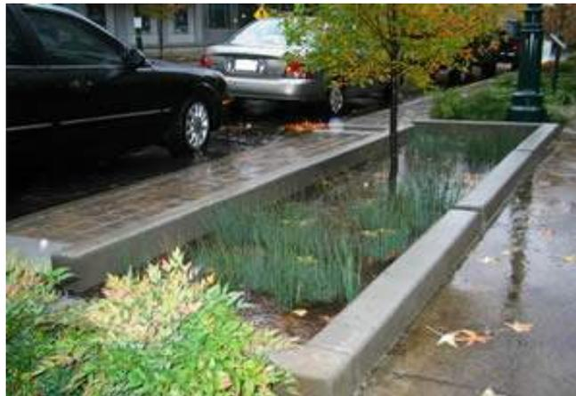
**Figure 9-A.2. Expanded Tree Pits**
