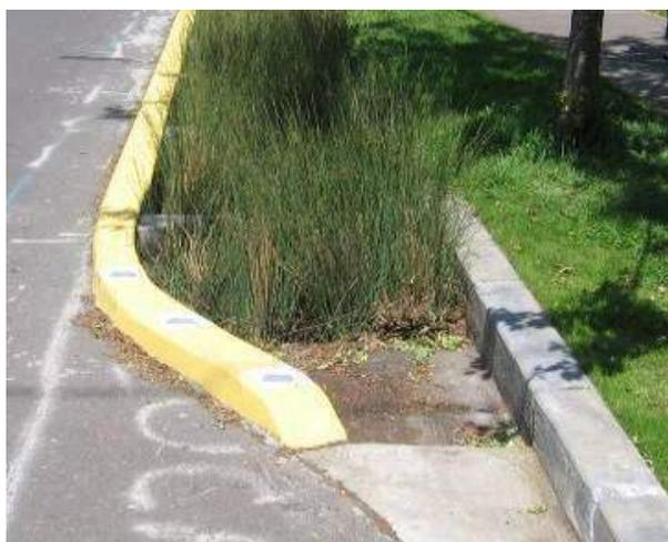
**Figure 9-A.3. Stormwater Curb Extensions**
