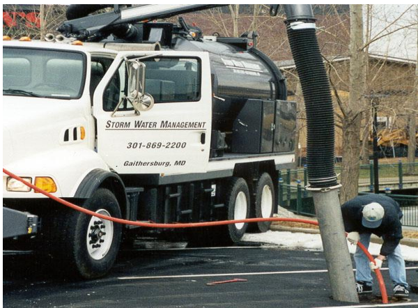
Figure 5: Vacuum truck and high pressure hose
