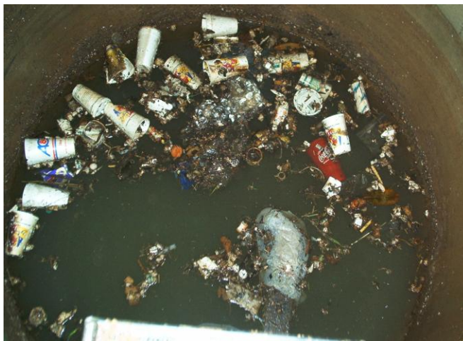
Figure 2: Storage manhole with floating debris and oils
