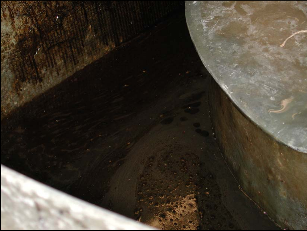
Figure 19. Outer chamber after 250 GPM test
