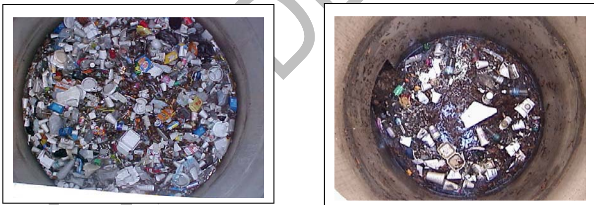
Figure 23 Gross Pollutants Captured in the CDS Units Sump
