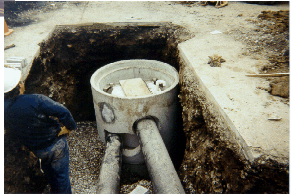
Stormwater Vortex Unit Installation
