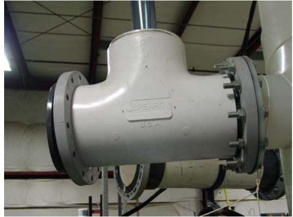
FD Outlet Into Test Tank
