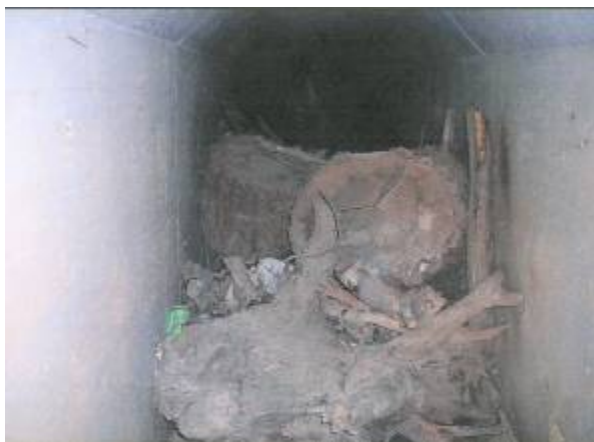
Figure 3-E.5. Clogged Storm Drains That Need to Be Cleaned Out
