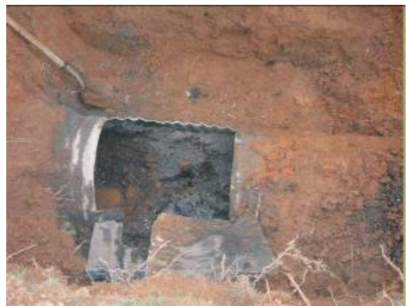
Figure 3-E.5. Clogged Storm Drains That Need to Be Cleaned Out
