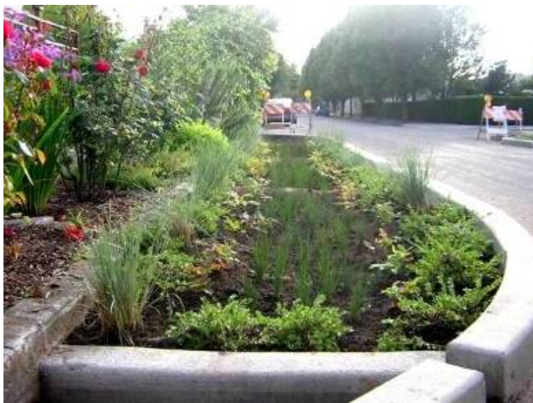
Figure 5-C.17. Bioretention Along a Green Street
