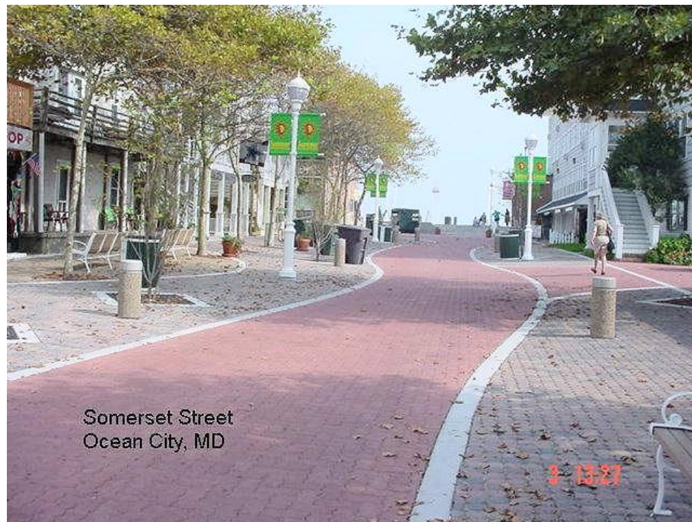
Figure 5-C.14. Permeable Pavers in Ocean City, Maryland
