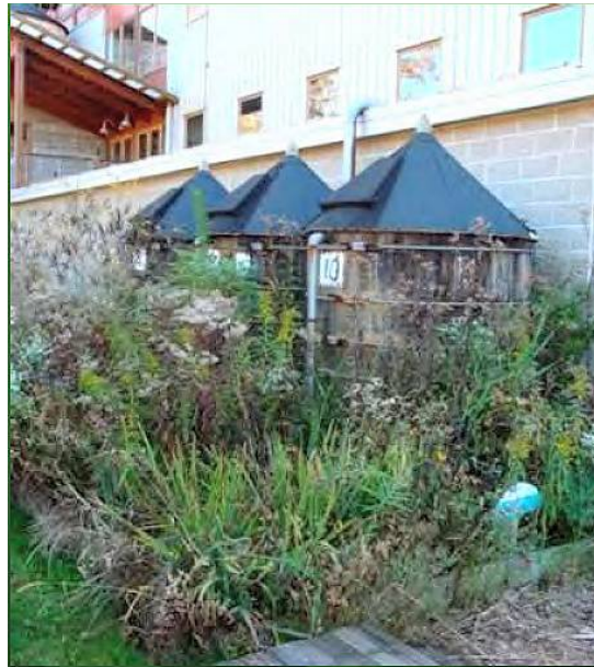
Figure 5-C.12. Rainwater Harvesting Cisterns
