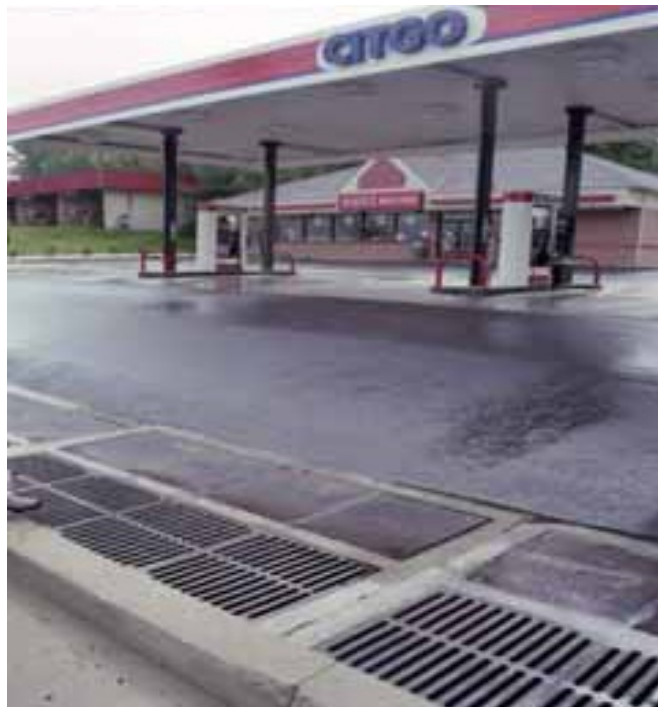
Figure 5-C.16. Delaware Sand Filter Under Grates Source: Center for Watershed Protection
