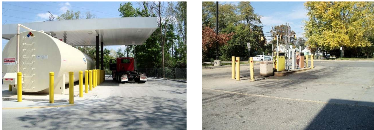
Figure 5-D.9. Covered vs. Uncovered Fueling Areas
