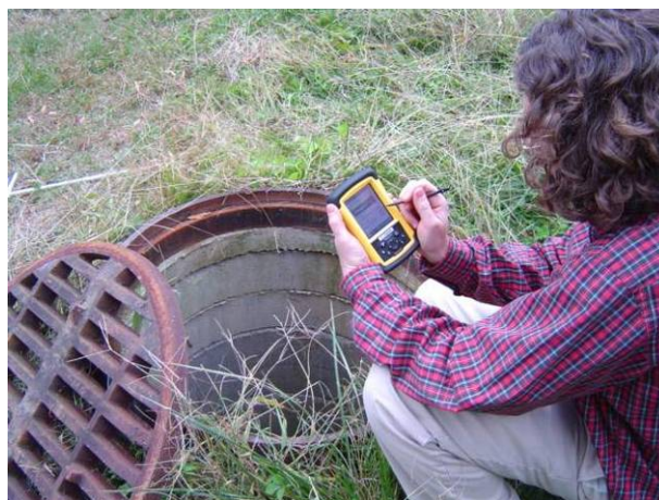
Figure 5-D.25. Storm Drain Inlet Inspection
