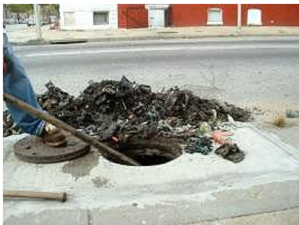
Figure 5-D.24. Catch Basin Cleanout
