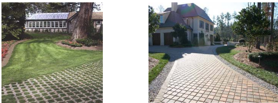
Figure 6.53. Alternative (Permeable) Driveway Surfaces
