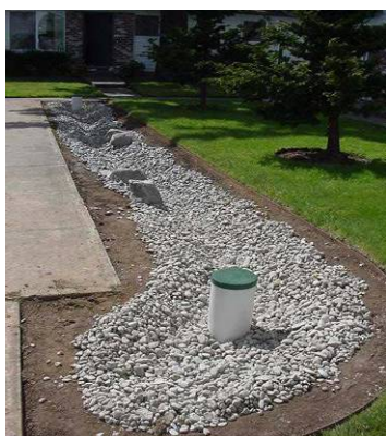
Figure 6.96. Infiltration Trench
