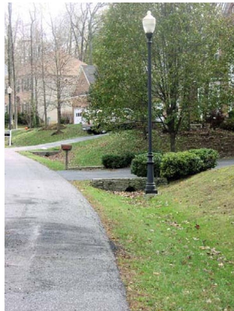
Figure 6.92. Subdivision Street Swale Drain.
