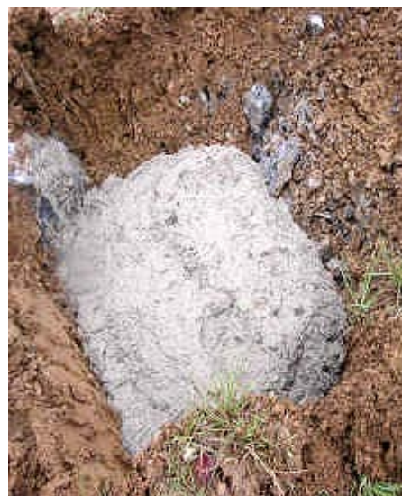
Figure 6-B.23. Grouting a Sinkhole
