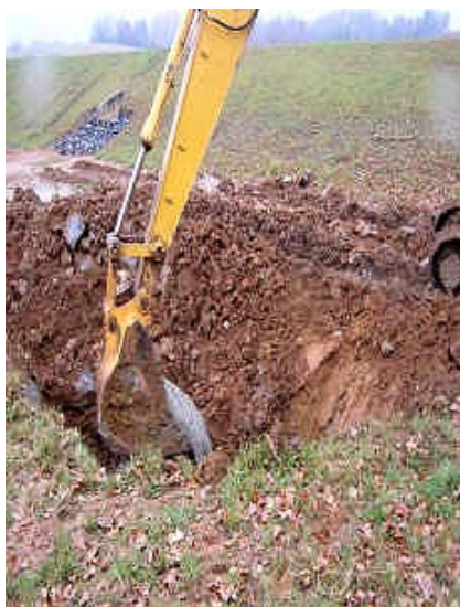
Figure 6-B.22. Sinkhole Remediation
