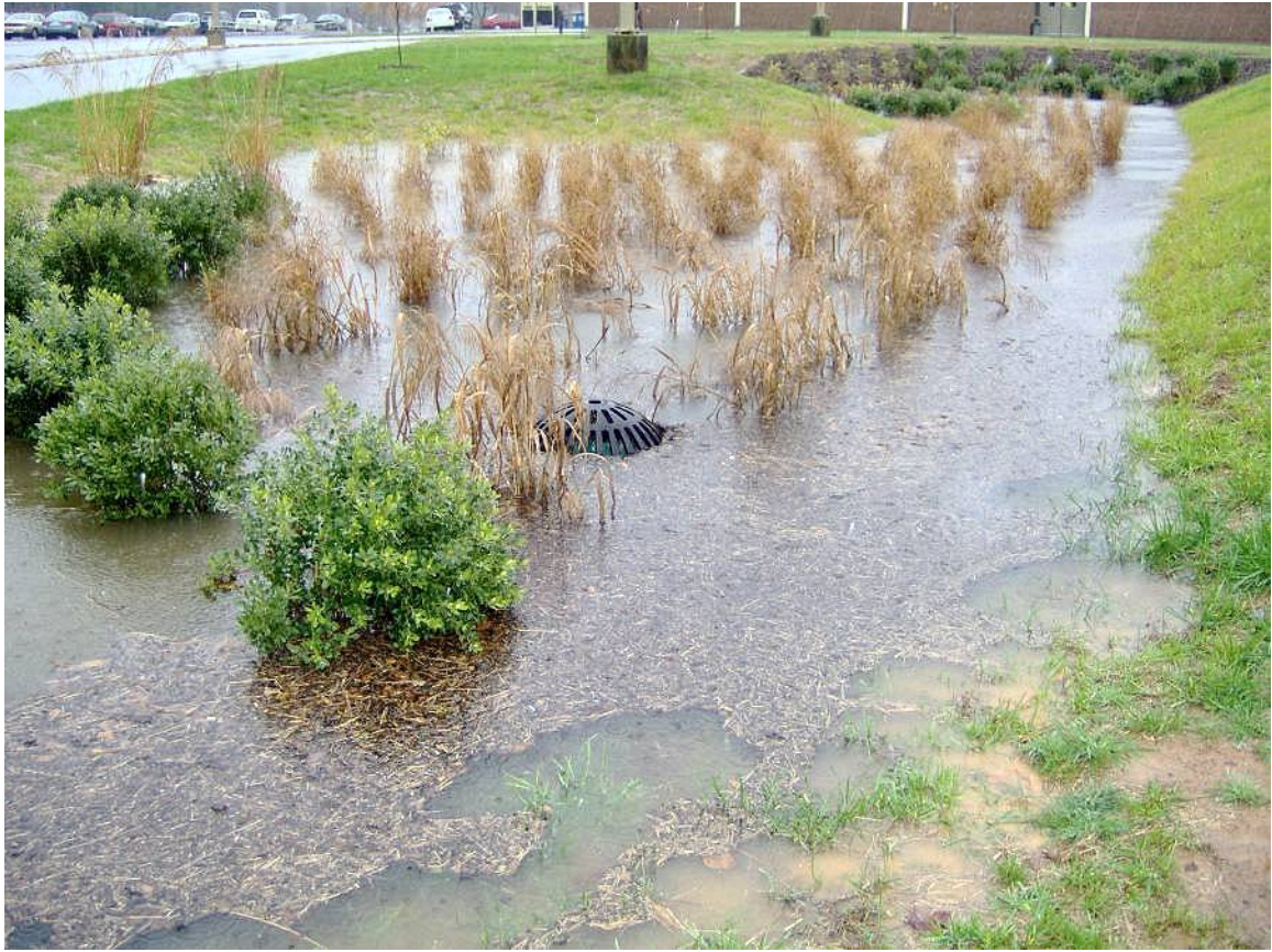
Figure 7-A.13. Charlottesville High School Bioretention Filter
