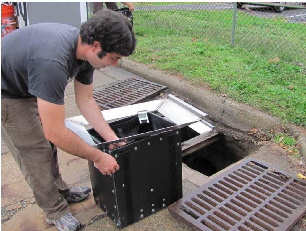
Figure 7-A.20. City Yard Catch Basin Filter Inserts
