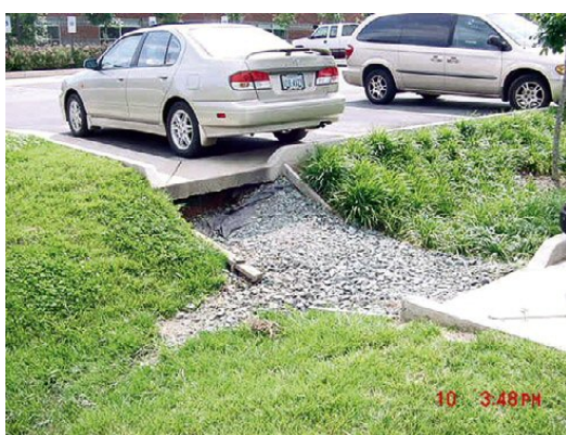
Curb inlets to bioretention swale have eroded.
