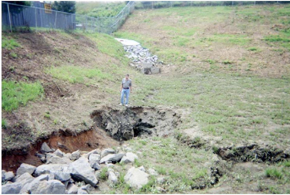
Figure 9.8. BMP Sinkhole Collapse
