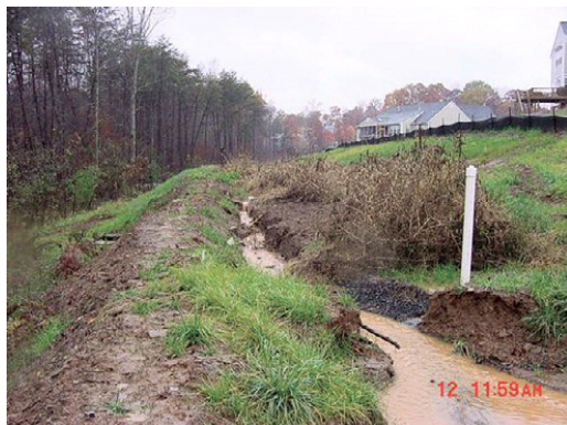
Bioretention swale clogged with sediment.
