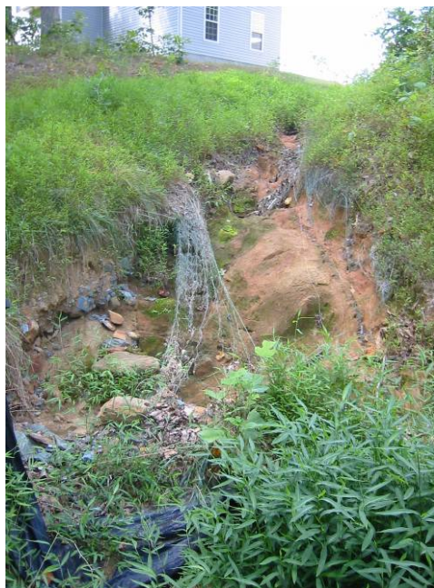
Figure 9.1. An unmaintained stormwater conveyance channel now generating sediment to the receiving channel (Source: CWP, 2009)
