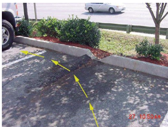
Site runoff bypasses bioretention swale.
