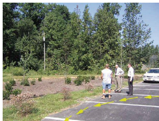
Some site runoff bypasses bioretention.
