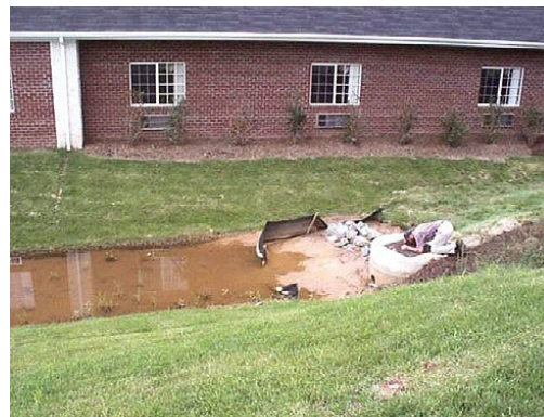
Bioretention area does not drain properly.
