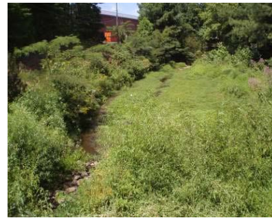
Sediment forebay filled in and became vegetated
