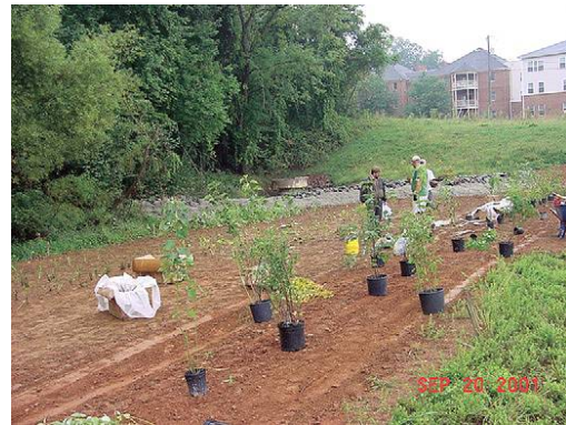
Planting Plan: Plants are being added to this regional basin to Enhance aesthetics and water quality functions.
