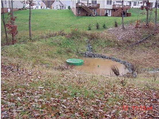
Not a Community Amenity: Unsightly basins in residential areas tend to become nuisances and generate complaints.
