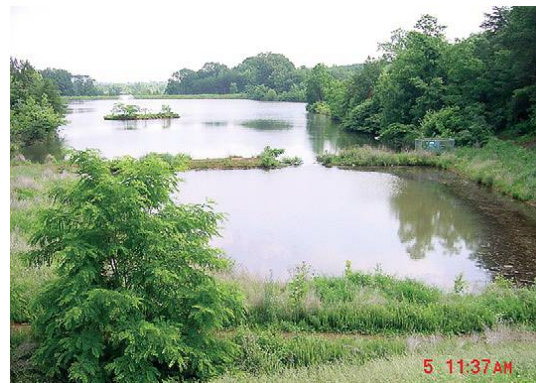
Pretreatment: Forebays and pretreatment cells help protect The main pond and ease future maintenance.
