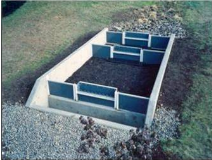
Photo: Compost Filter; courtesy Stormwater Management Inc.
