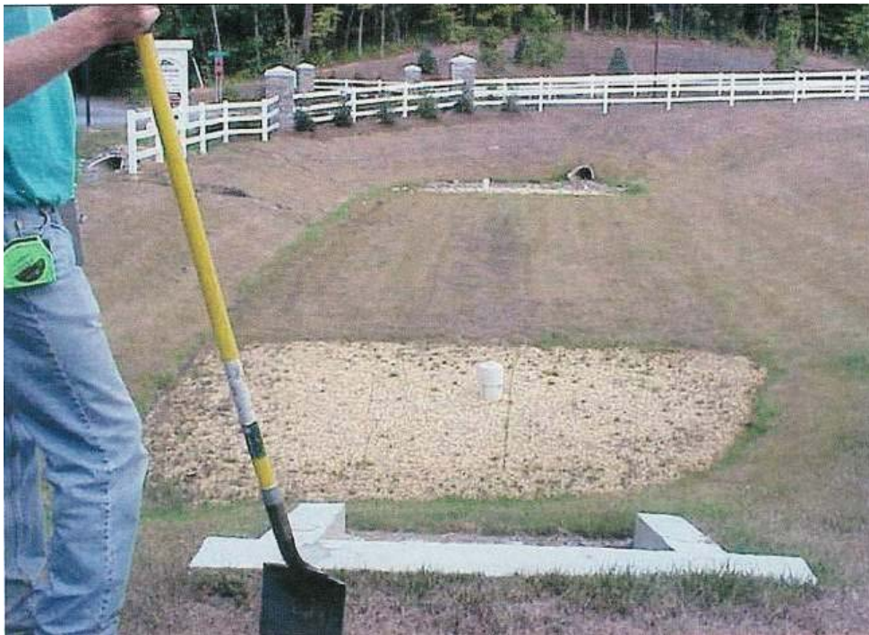
Figure 12.5. Hybrid Sand filter in a Detention Basin
