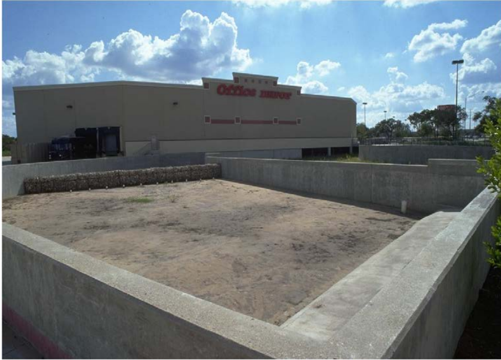
Figure 12.6. Austin Surface Sand Filter
