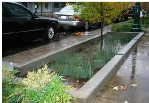
**Figure 9-A.2. Expanded Tree Pits**
