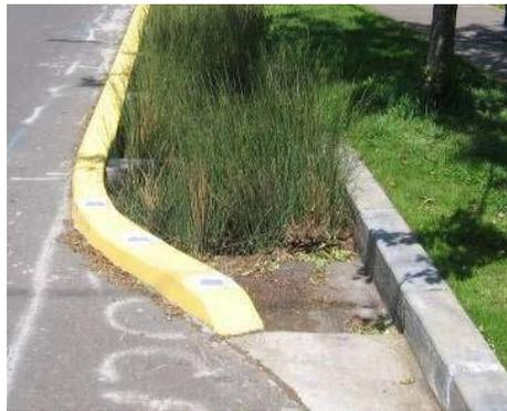
Figure 9-A.3. Stormwater Curb Extensions
