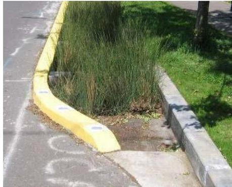
Figure 9-A.3. Stormwater Curb Extensions
