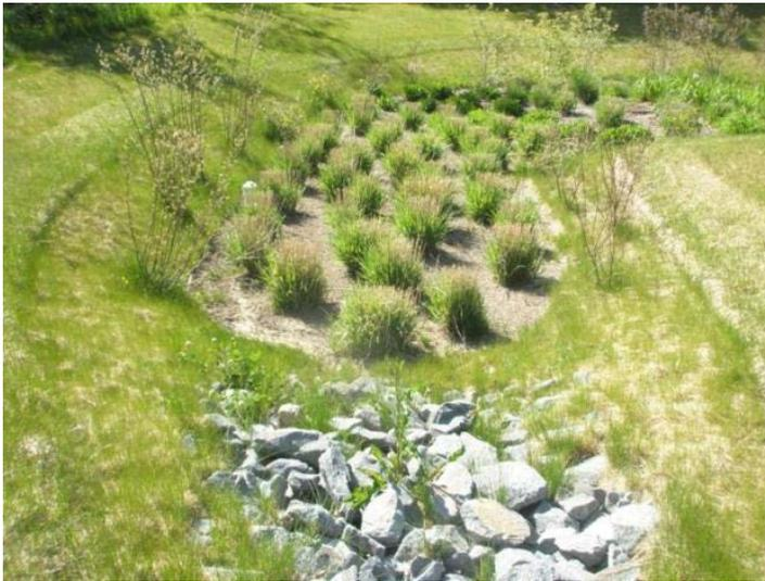
**Figure 9.1. Typical Bioretention Filters**
